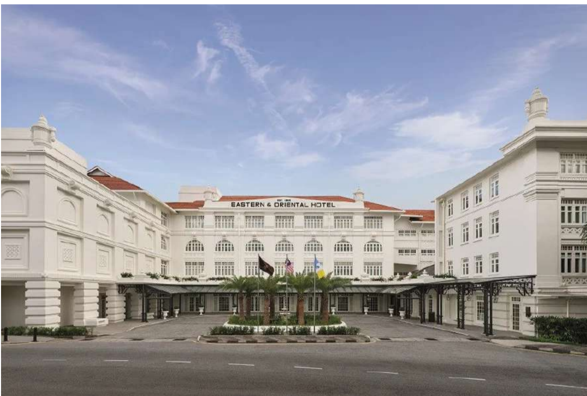
The E&O's Heritage Wing facade.
