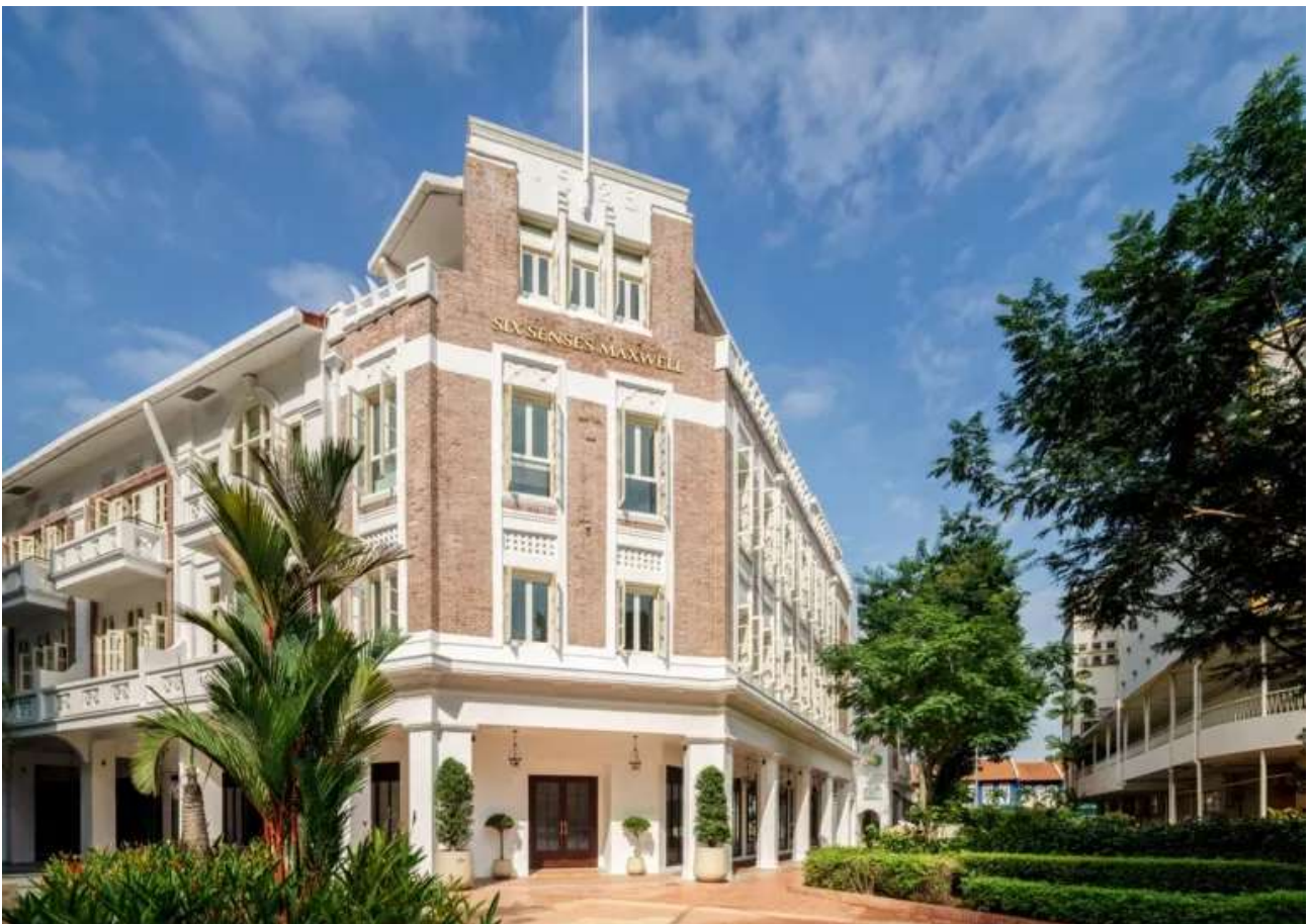
The Six Senses Maxwell hotel occupies former 19th-century shophouses in Singapore's Chinatown. (Photo courtesy of Six Senses)
